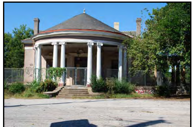
Figure 35: Kriegshaber House, 292 Moreland Avenue
