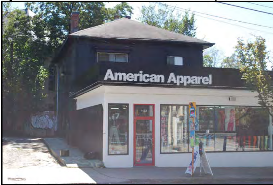
Figure 41: 1133 Euclid Avenue (Former Moreland Military Institute Building)
