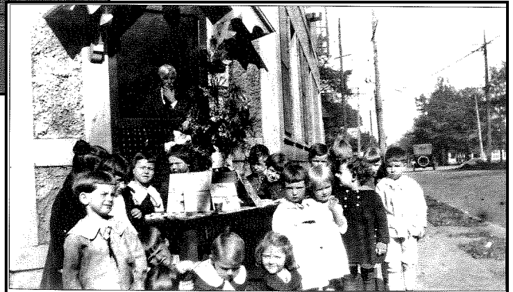
Figure 16: 1916 Photograph of the Church of the Epiphany. An automobile heading north on Moreland Avenue is visible.
